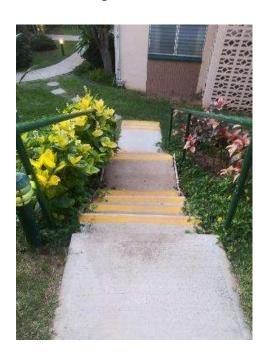
The instant installed stairs in the hill by building #6 were not built to code so the Board of Directors elected to remove the stepping stone steps and replaced it with a cement stairway to bring it up to code with two handrails.
