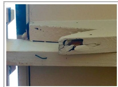
Termite damage
